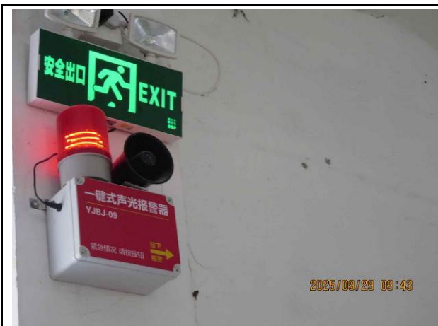
Fire alarm testing
