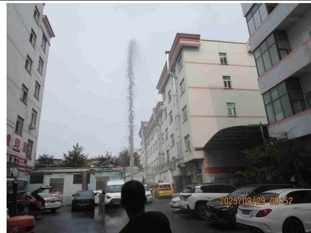
Test for fire hydrant
